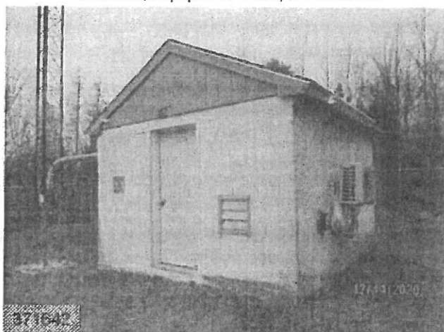
Shelters, Equipment Pads, & Platforms
