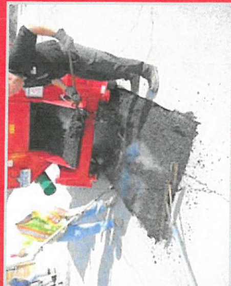
COAT ASPHALT WITH REJUVENATOR
