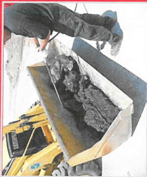
COAT ASPHALT WITH REJUVENATOR
