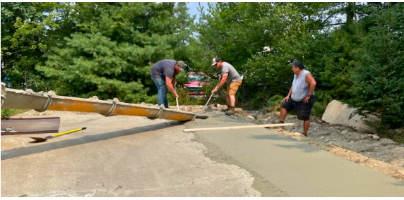
An extension was added to the concrete surface at the Transfer Station to improve safety while maneuvering the forklift.
