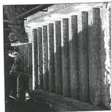
6 RUN OF STAIRS EXISTING APPROXIMATE VIEW NORTH
