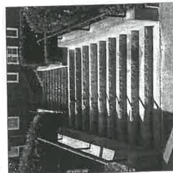
8 RUN OF STAIRS EXISTING APPROXIMATE VIEW SOUTH
