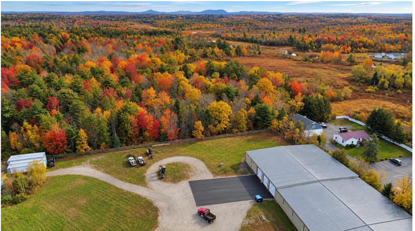
Approach to the future courthouse site during construction off the Merrill Lane traffic light.
