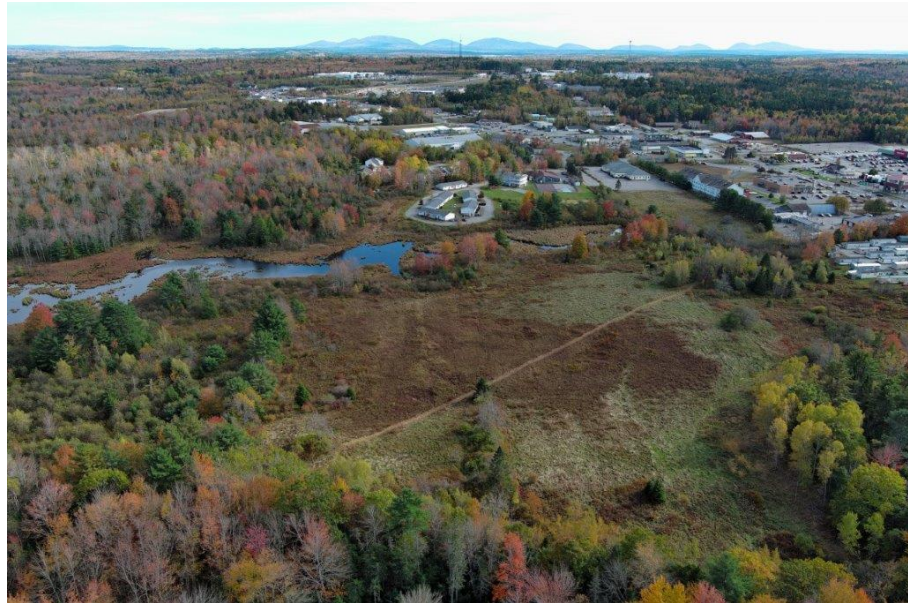
Merrill Lane corridor near High Street. City of Ellsworth photo, published October 2025.
