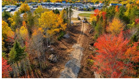
Aerial view of the road corridor during clearing. Photo supplied for this memo.
